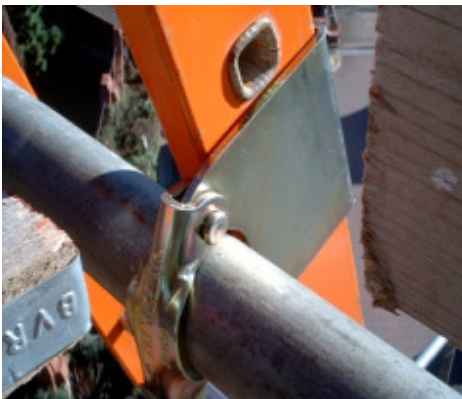
Ladder Coupler Fixing
